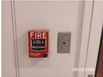
Fire Alarm Manual Station
