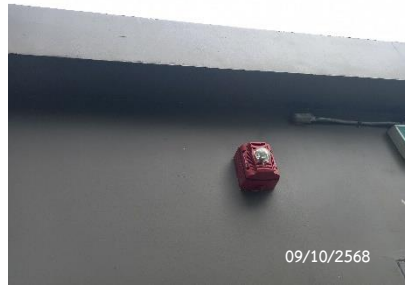
Indoor Selectable Output Speaker
