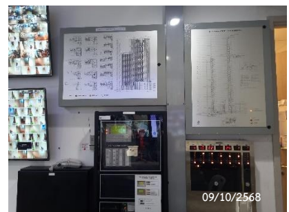
Graphic Annunciator Fire Alarm System
